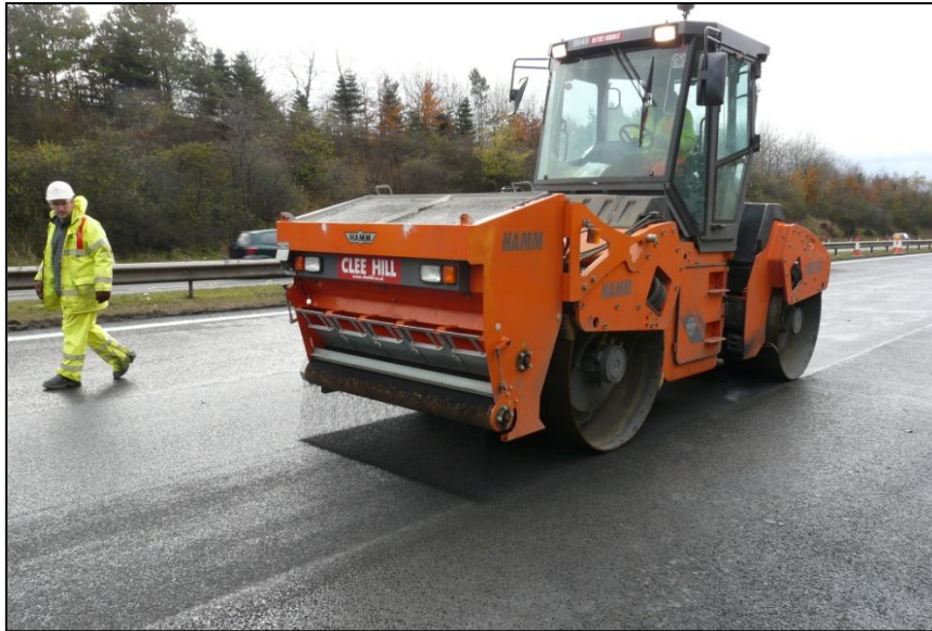
Figure 4.4 Applying grit to newly-laid SMA on the M8 trial site
