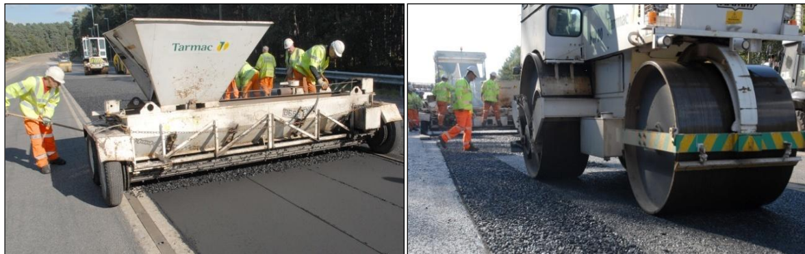
Figure 4.1 The spreading (left) and rolling (right) of chippings on the HRA section of the TRL test track
